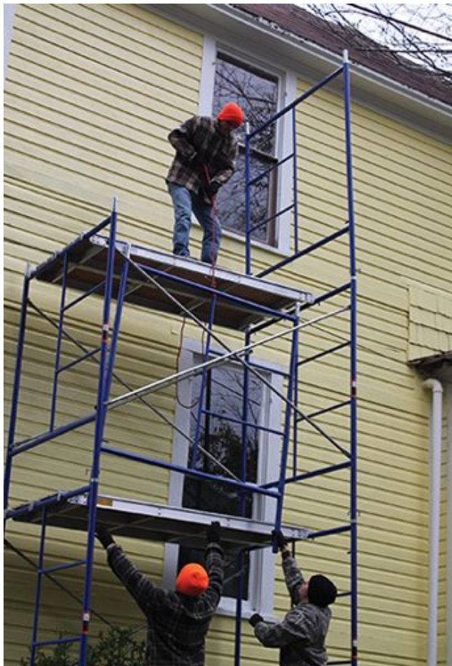
Scaffolds to Provide Access
